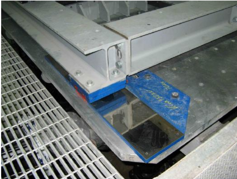
Fig. 11.22: Detail of the PTFE flat sliding bearing
