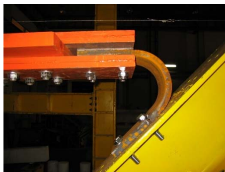
Figure 3.2: U-PLATE INERD CONNECTION
