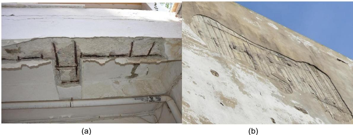
Figure 3.2: (a) Concrete's delamination at a 1st floor balcony (b) Concrete's delamination of a wall in the building's rear view
