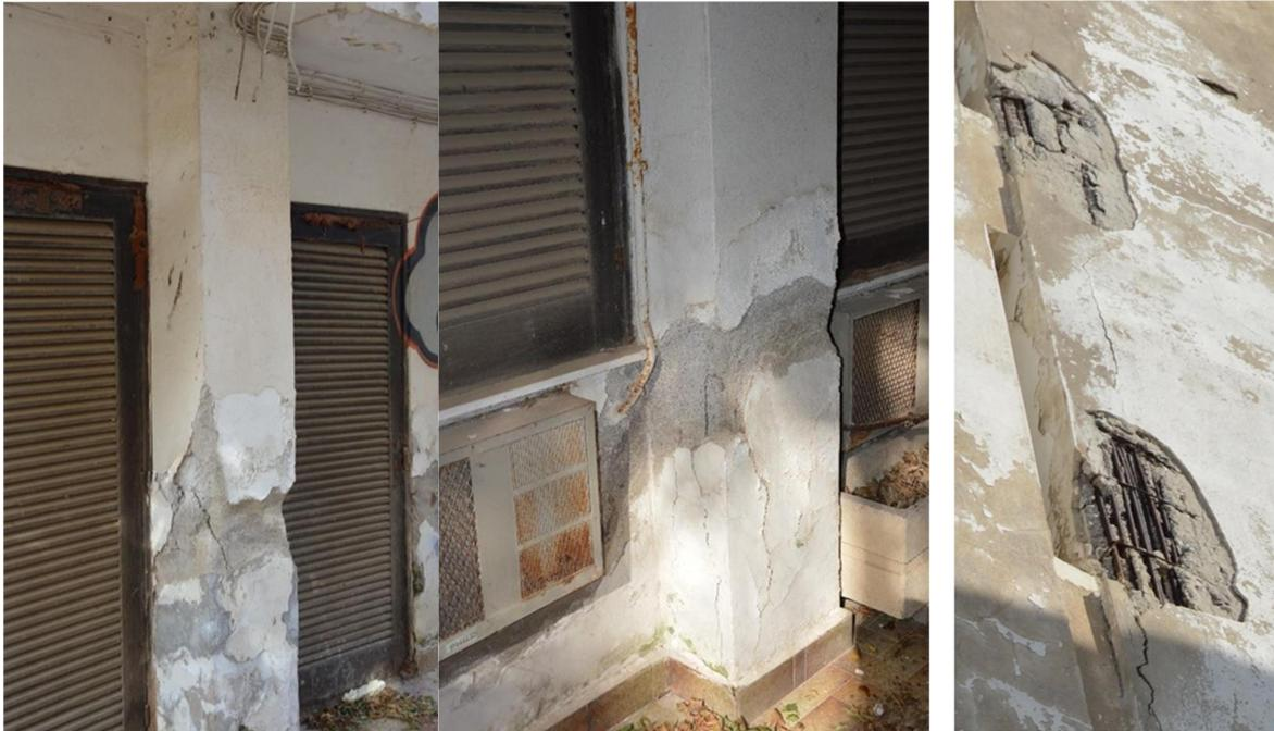
Figure 3.3: Concrete's fracture of a wall in the building's rear view, Concrete's degradation of a column at its base without evident reinforcement buckling while at its top a delamination is noted
