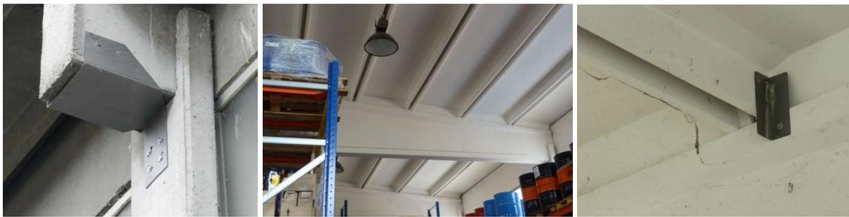
Figure 6.2: Details of connections between structural elements and structural/non-structural elements.
